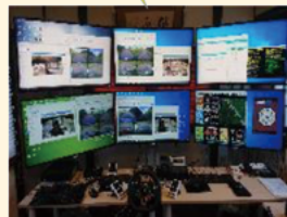
Remote monitoring and inspection room
