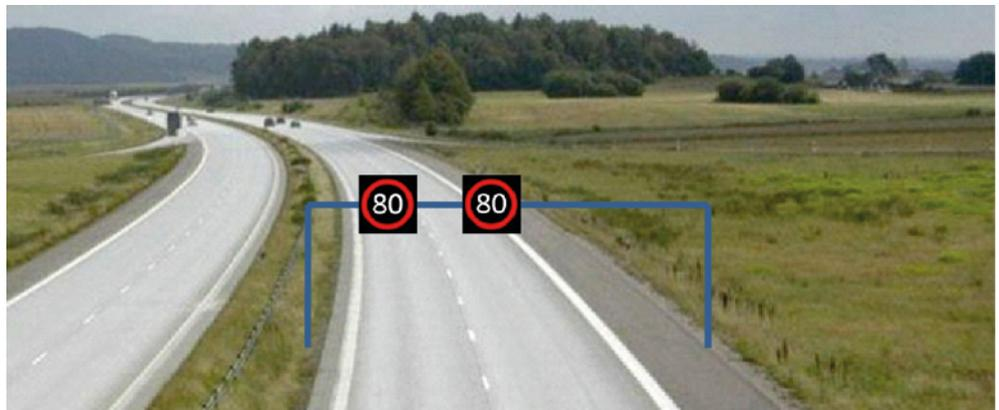
Figure 55: **Portal mounted VSL signs on motorway, one speed limit sign integrated in VMS according to CL&FR5**
