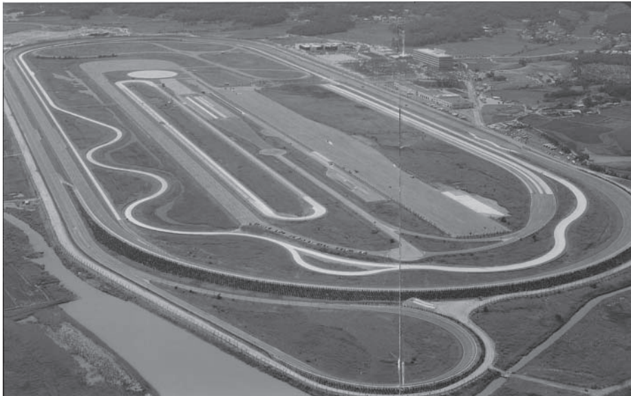
Figure 15.9 View of Hyundai Research Centre at Namyang
