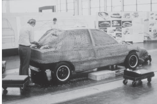
Figure 4.8 Claying up armature to hardpoints
