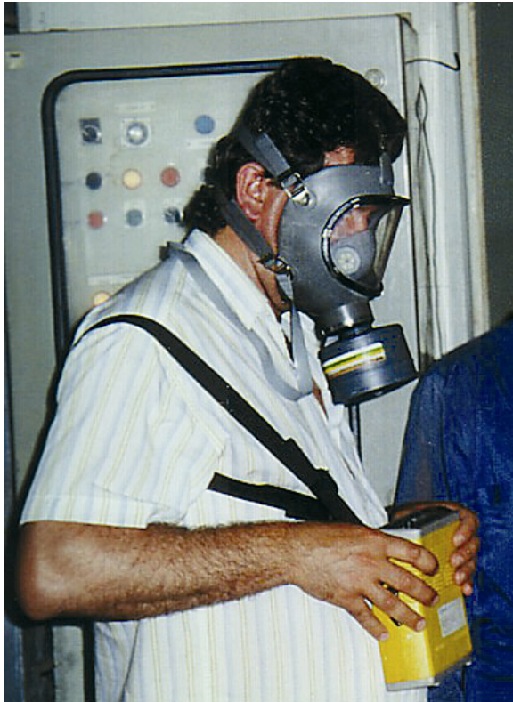
Figure 3.2 Hydrogen sulphide is often present in the influent to treatment plants, especially in case of pressurized sewers. It is very toxic and can result in casualties of personnel which do not take the necessary precautions. The picture shows measurement in the pumping station with high hydrogen sulphide concentration in the air (photo: M. Henze).
