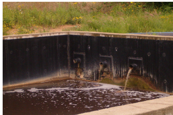
Figure 3.6 Collection and storage of leachate at sanitary landfill of Sarajevo in Bosnia and Herzegovina (photo: F. Babić)
