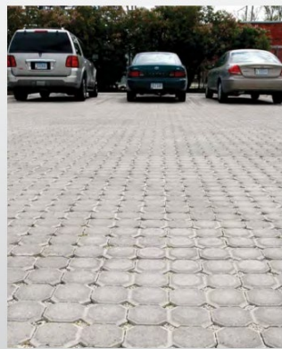
Rainfall soaks through permeable pavement and into the ground below in this parking area in west Des Moines, Iowa.
