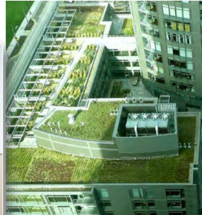
A green roof absorbs rainwater, reduces energy costs and offers wildlife habitat in urban Portland, Oregon.
