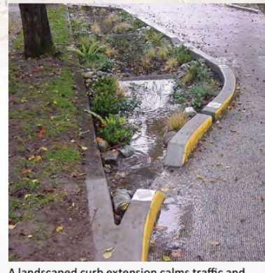
A landscaped curb extension calms traffic and captures and infiltrates street runoff in Portland, Oregon.
