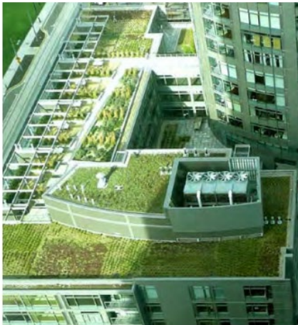
A green roof absorbs rainwater, reduces energy costs and offers wildlife habitat in urban Portland, Oregon.
