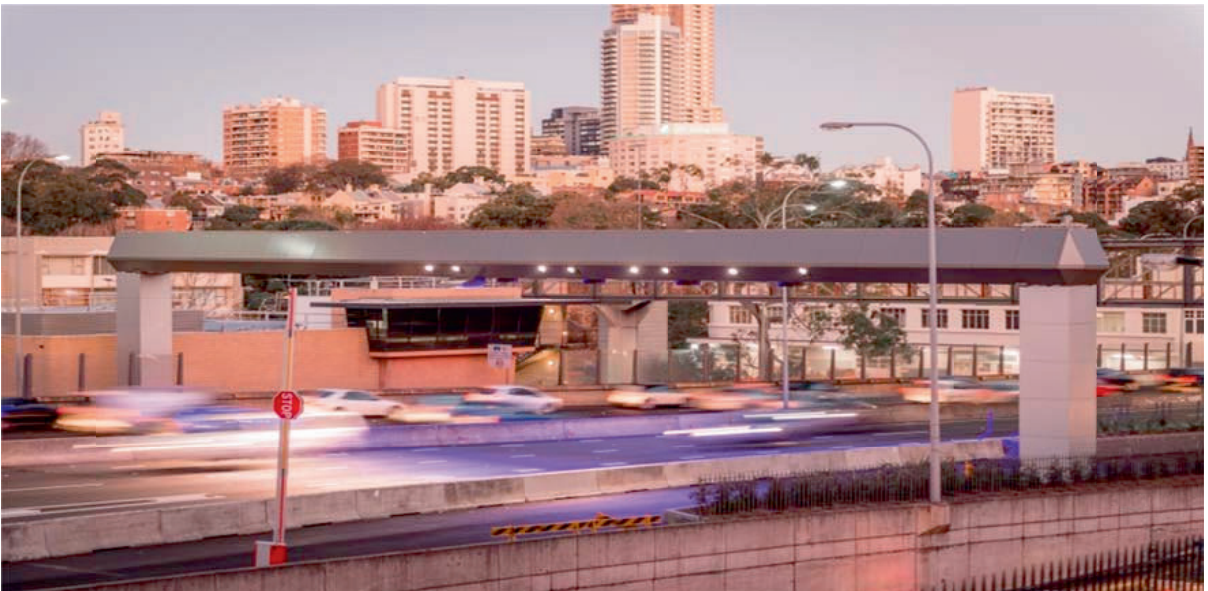
Figure 12 Installation of a gantry for an electronic toll collection system
