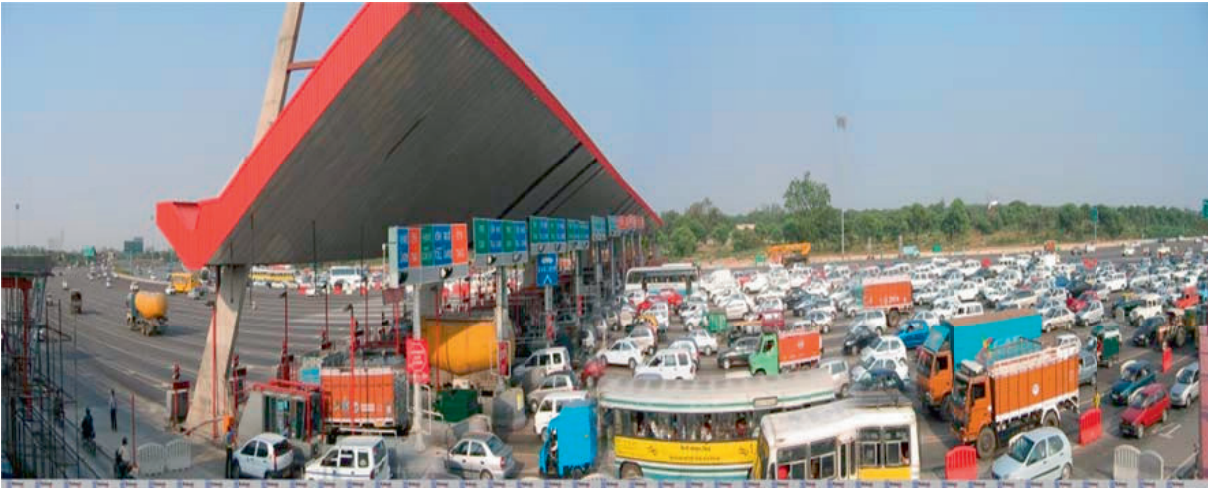
Figure 11 Installation of a toll plaza for a manual toll collection system
