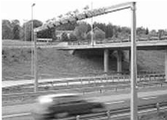
Figure 7.6 Multilane no-stop tolling. (Source: Q-Free.)
