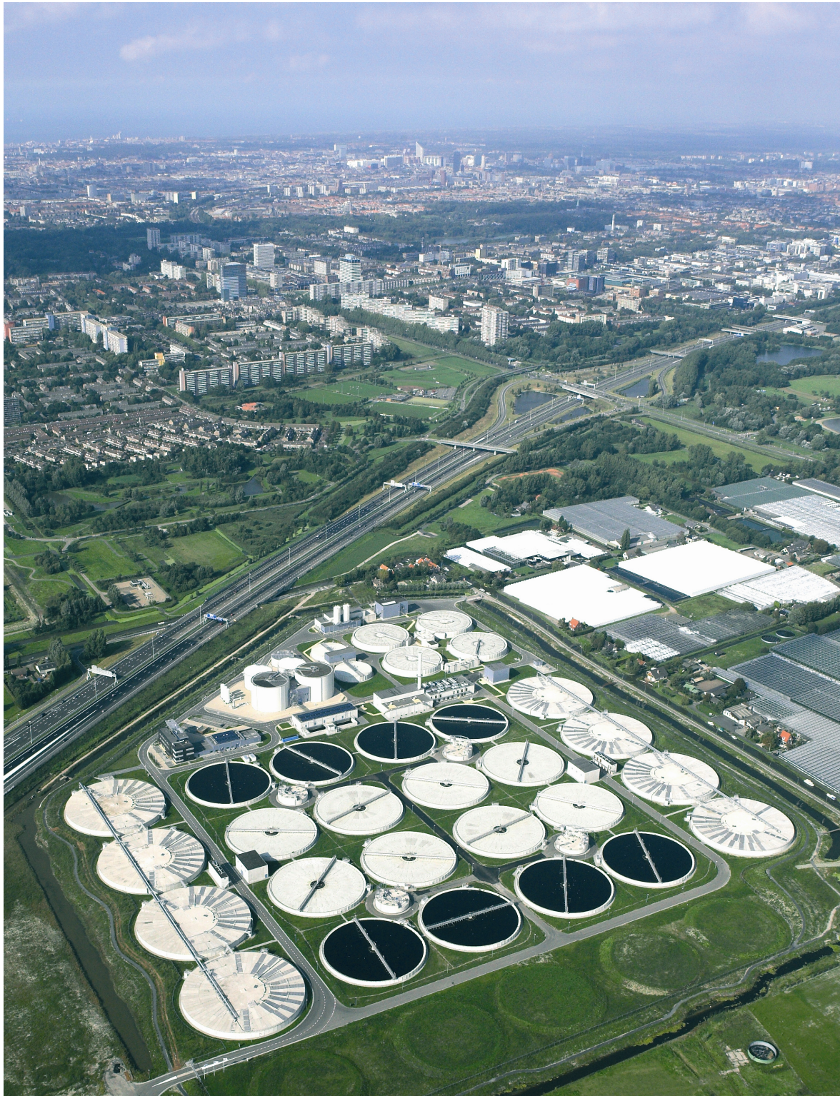
Wastewater treatment plant Harnaspolder is a large plant (1.31 million P.E.) collecting wastewater from the Den Hague region. This is the first plant in The Netherlands whose construction was financed by a public-private partnership (photo: Aeroview-Rotterdam provided by courtesy of Delfluent B.V.)
