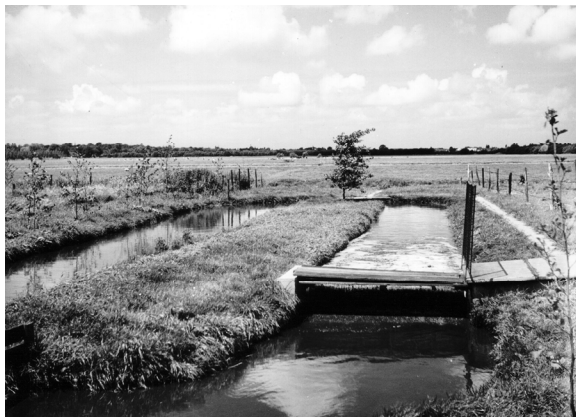
Figure 1.2 The first (pilot) application of Pasveer ditch system (1954 Voorschoten, The Netherlands). The plant capacity was 400 P.E. and 40 m 3 /h at dry weather flow (photo: van Lohuizen, 2006)
